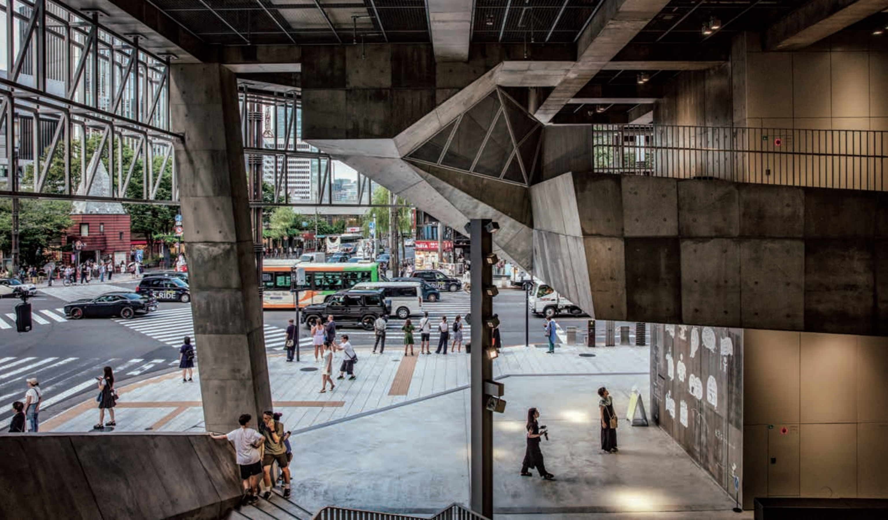
The open structure of Ginza Sony Park beckons passersby to interact with the space and linger, turning an everyday stroll into a unique experience.
